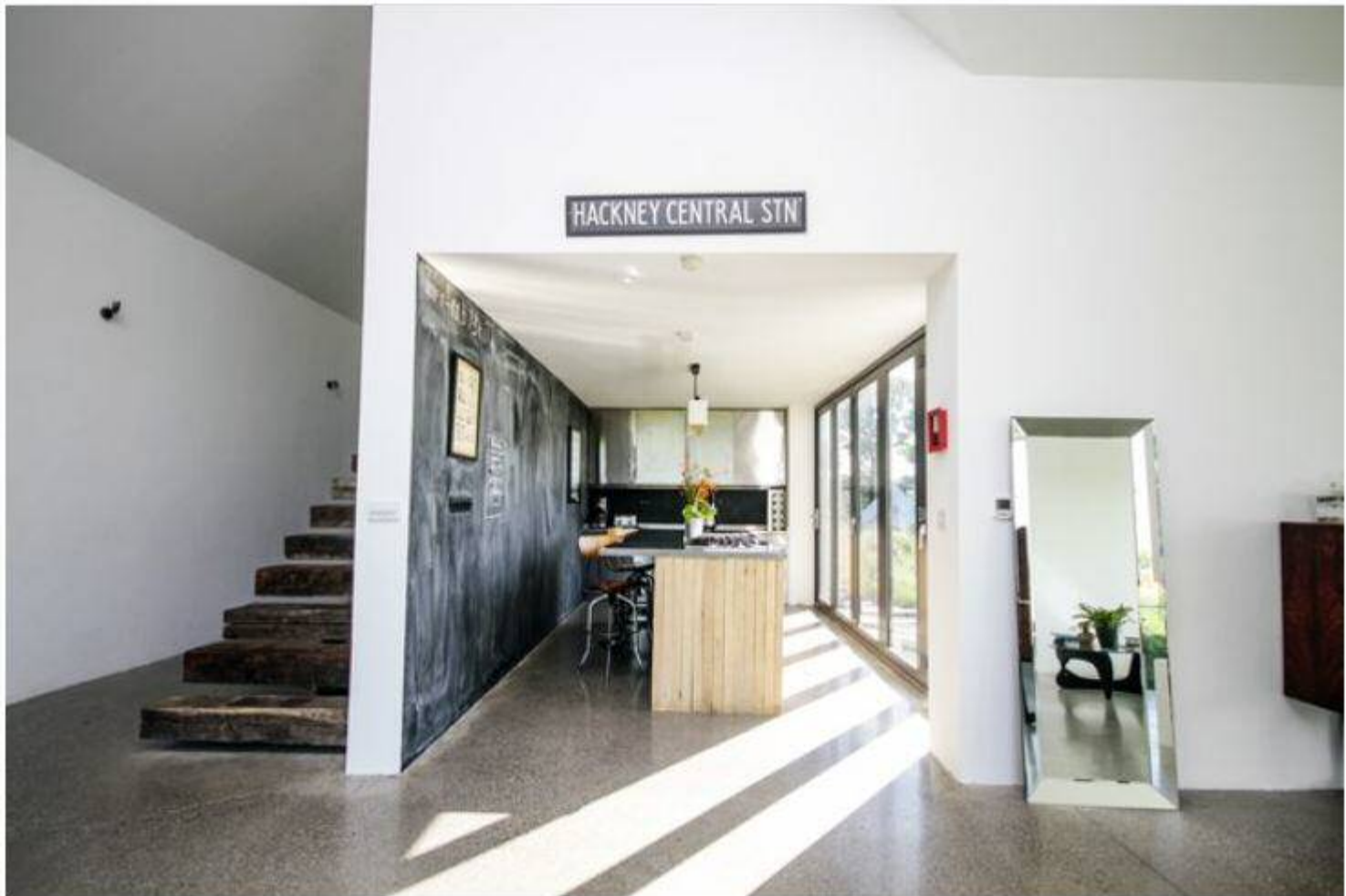
The staircase is made of old railway sleepers.
